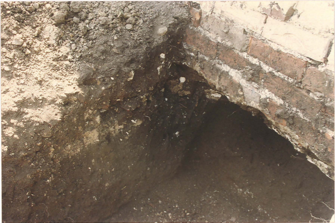
PI. 13 Trench M. The brick foundations of the extension cover vestigial courses of a chalk foundation; the mortar layer alongside the wall is fill of the earlier foundation trench, with clay above it filling the brick foundation trench. The thick brown clay layer is bank material alongside the linear depression. Looking SW.
