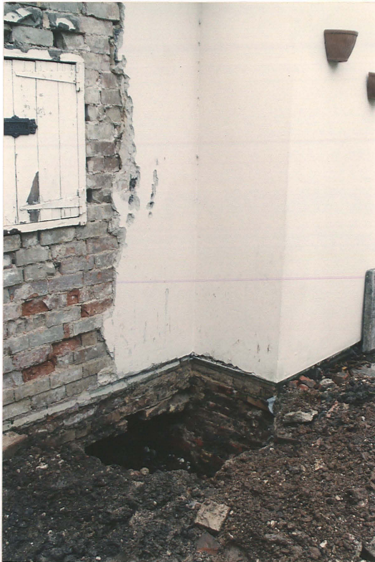
Pl. 2 Trench A, for underpinning existing extension to Wyham Grange (looking SE).
