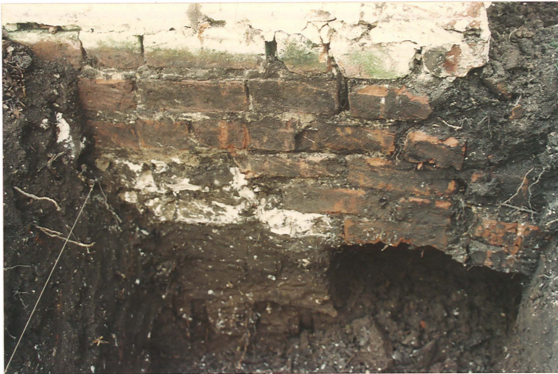
Pl. 12 Foundation courses at the NE corner of the extension (Trench L). The existing brick extension over-rides chalk block foundations of an earlier structure. Looking west.
