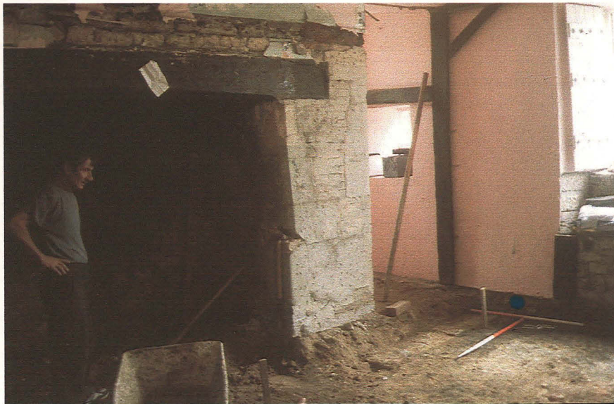
Plate 2 - Exposed fireplace in Room 8, looking southeast
