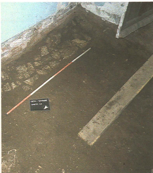
Plate 6 - Phase 1 foundation wall (014), looking southeast
