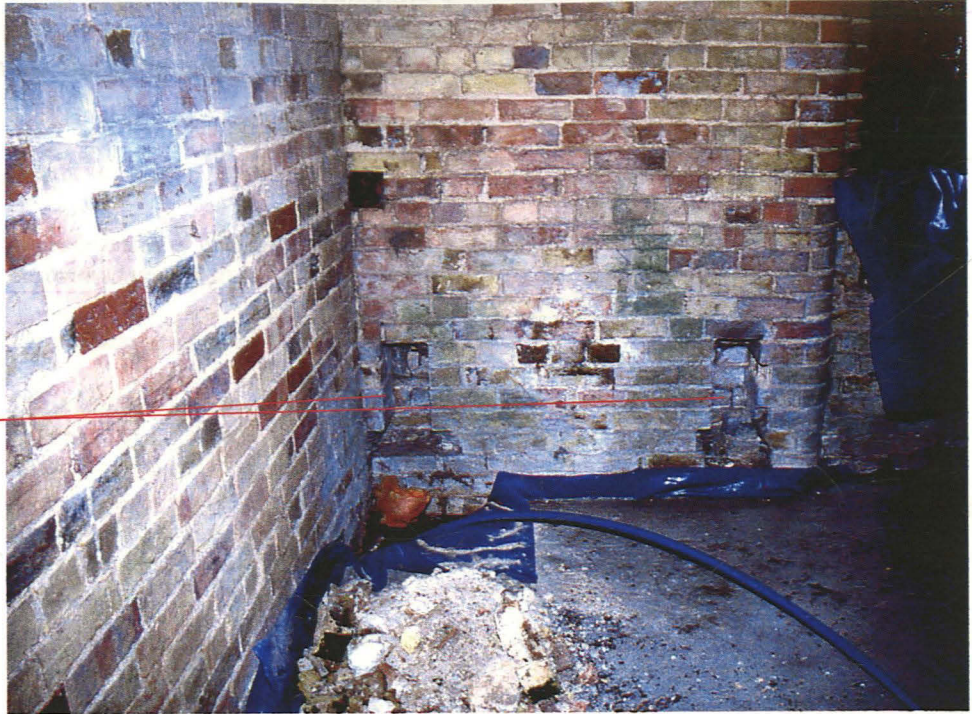
Plate 6 Machinery voids seen in northeast interior wall
