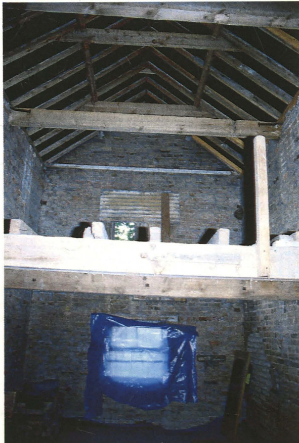
Plate 7 Interior view of first floor rafters and roof trusses
