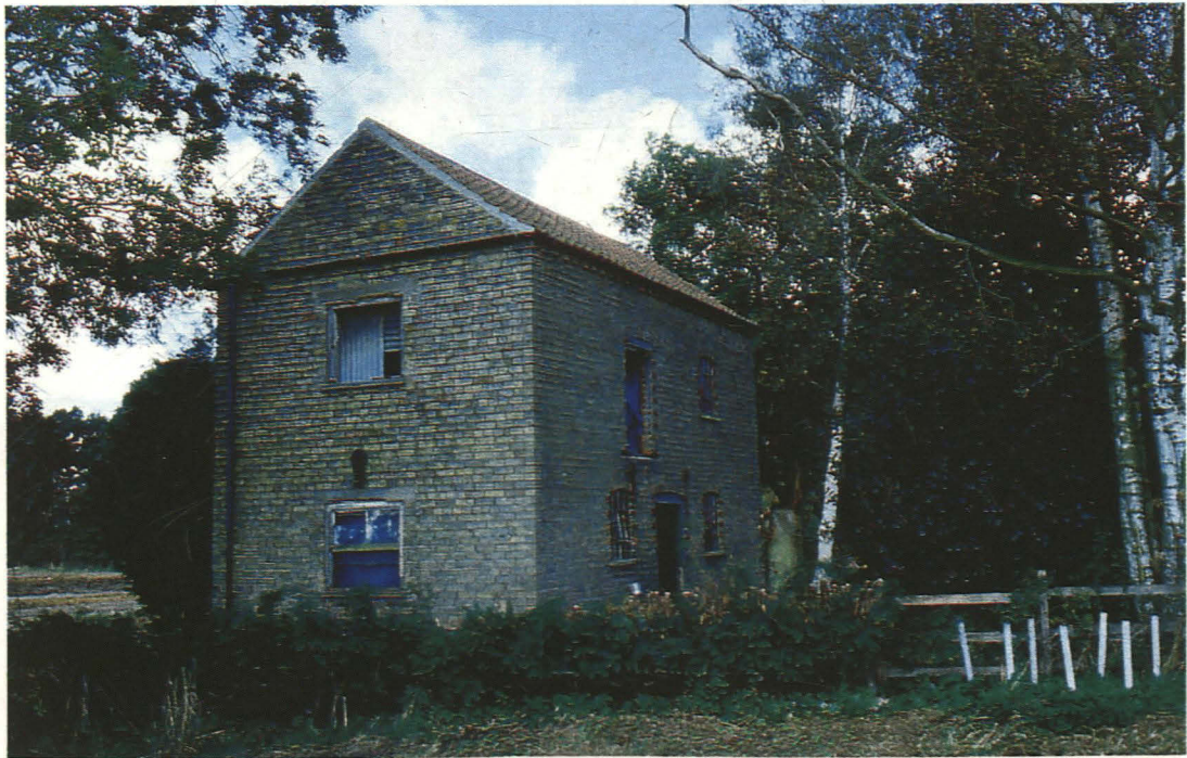
Plate 2 Southeast façade of Old Steam House
