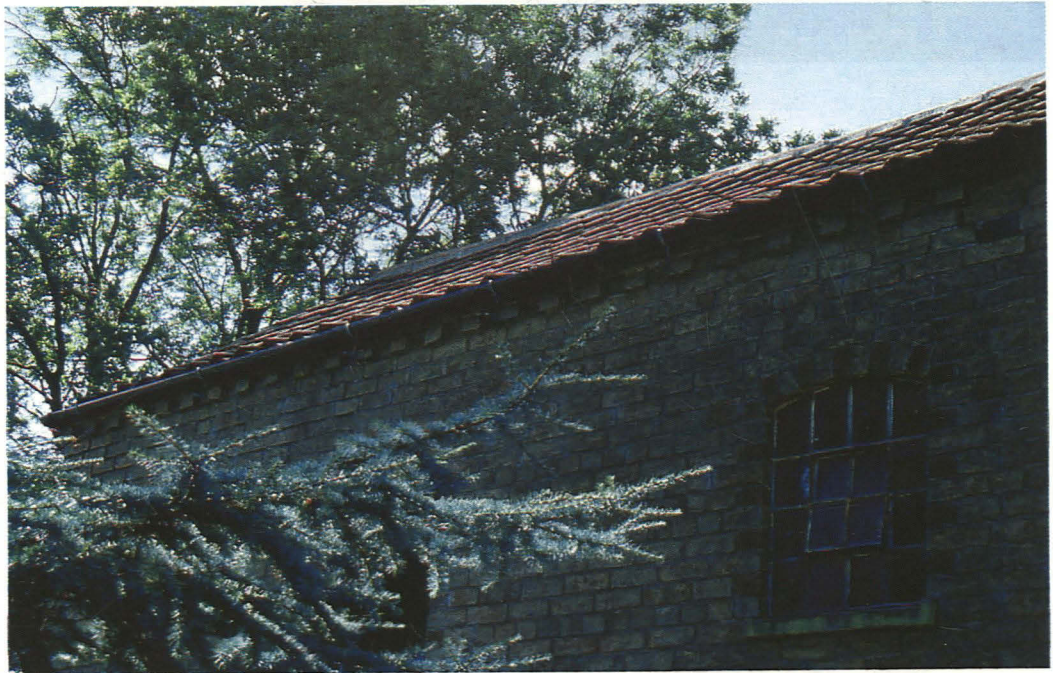
Plate 5 Brick patching denoting former entrance and window in southwest façade
