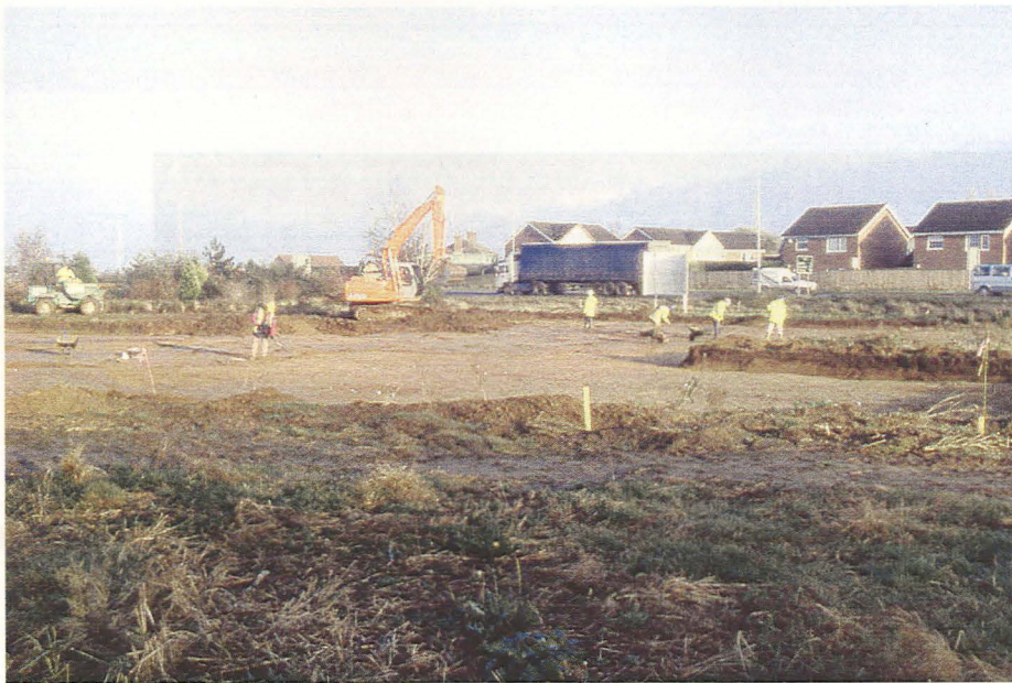
Plate 1 General view of Excavation Area, looking East
