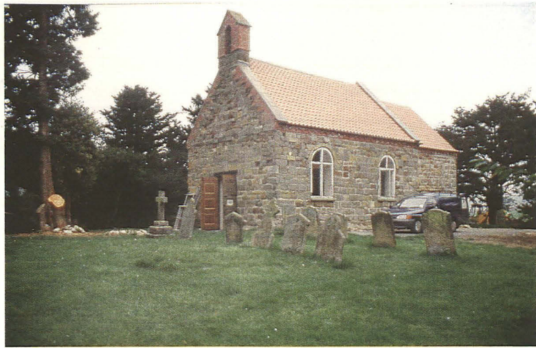
Plate 1 - St. Andrew's church, from the southwest
