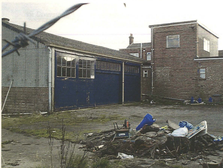
Plate 3 - The rear of the development area showing the building to be demolished, looking southeast
