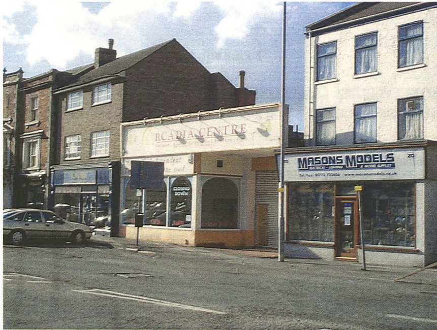
Plate 1 - General view showing the frontage of 18-19 New Road, looking northwest
