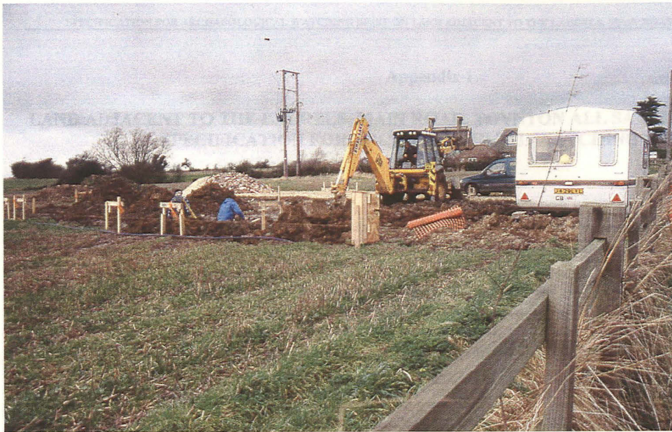
Plate 1 General view of site, looking northwest
