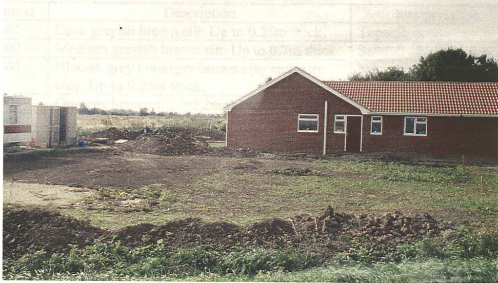
Plate 1 General view of the development site showing completed bungalow on Plot 2 and area of Plot 1 in the foreground. Looking southeast.
