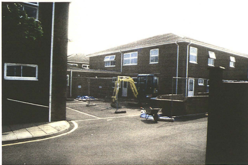
Plate 1 - General view of the development area, looking southeast
