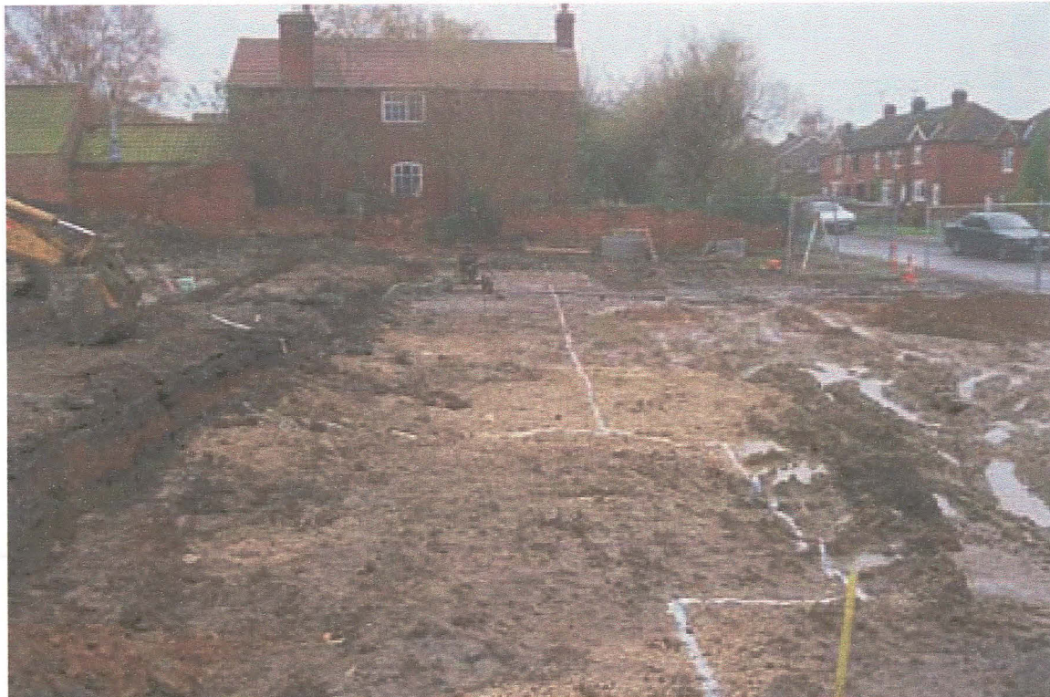
Pl. 2 House Plots 1-5, during excavation of foundation trenches (looking south).
