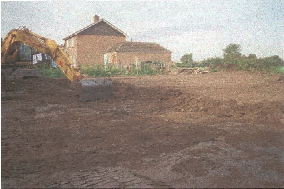
Pl. 7 House Plots 6 and 7, during topsoil removal (looking south-east).
