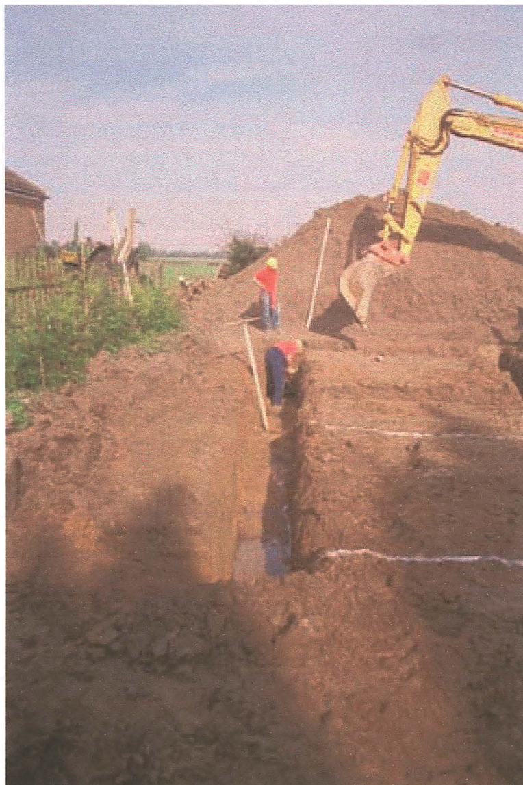
Pl. 8 Excavation of foundation trenches on Plot 7 (looking east).
