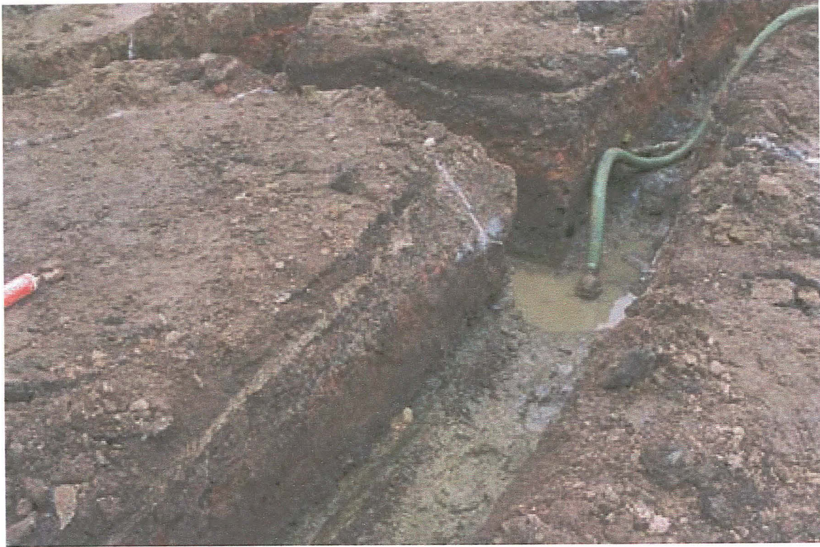
Pl. 3 A series of yard surfaces of asphalt, ash, gravel and brick rubble covered most of House Plots 1-5.
