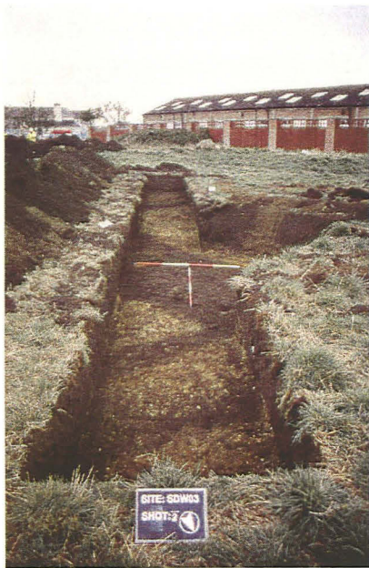
Plate 5 General view of Trench 5, looking southwest.
