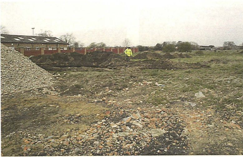
Plate 1 General view of the site, looking northwest.
