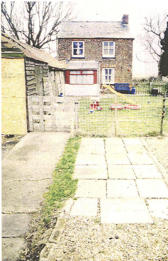
Plate 3 Southwest elevation, looking northeast
