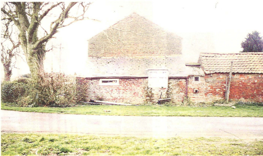
Plate 5 Northwest elevation, showing extension and additional outbuildings, looking north
