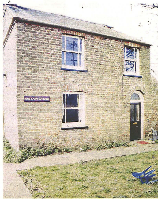
Plate 2 Northeast elevation, looking west
