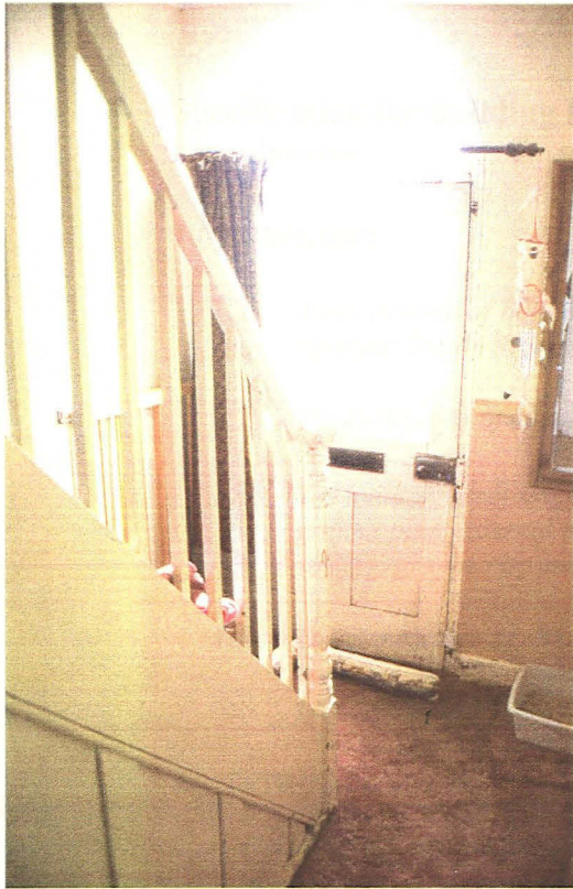
Plate 8 Hallway and simple square baluster, looking north
