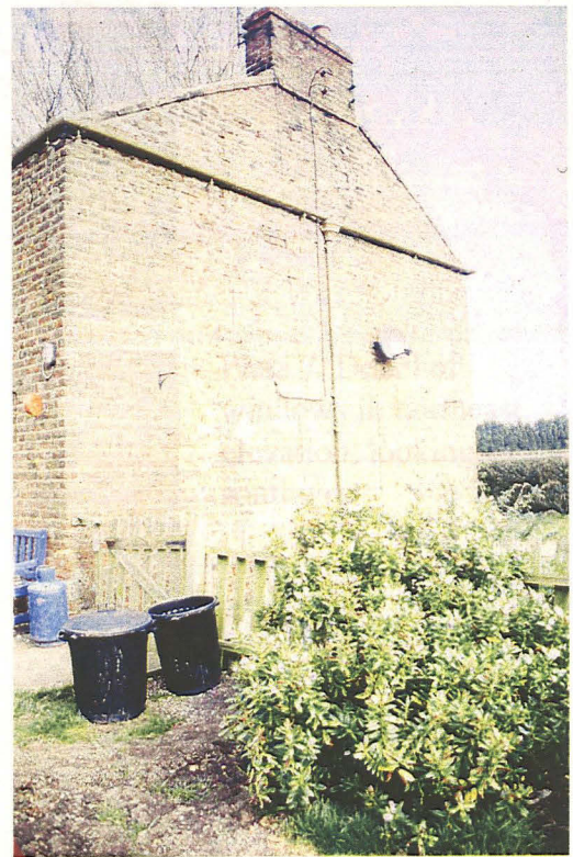
Plate 4 Southeast elevation with chimney in gable, looking north
