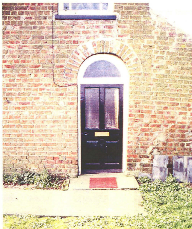
Plate 6 Details of front door, with lean to extension, looking southeast
