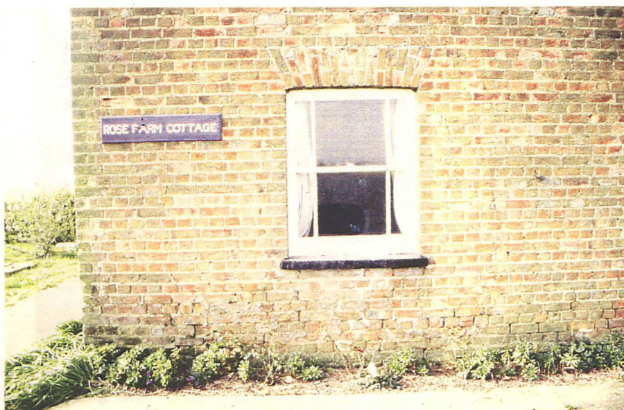
Plate 7 Detail of windows in northeast elevation, looking southwest
