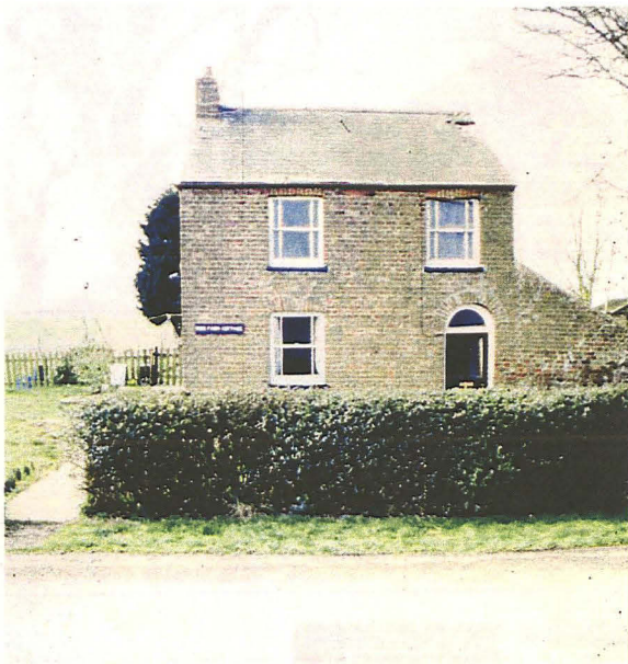
Plate 1 Northeast facing elevation, looking southwest
