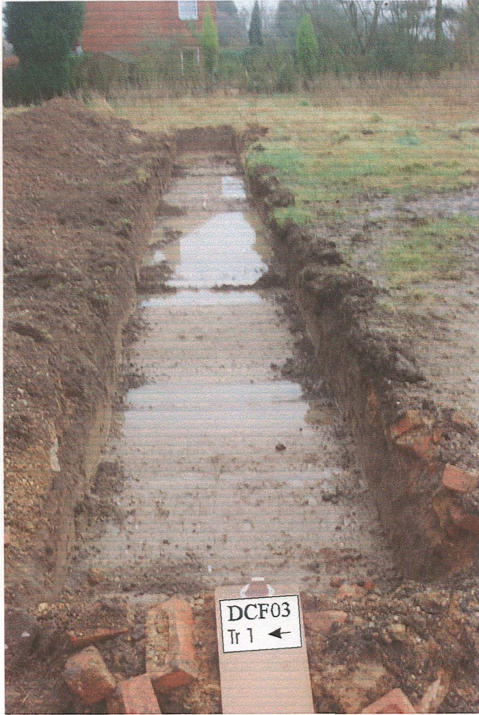
Plate 1. General view of Trench 1, facing east
