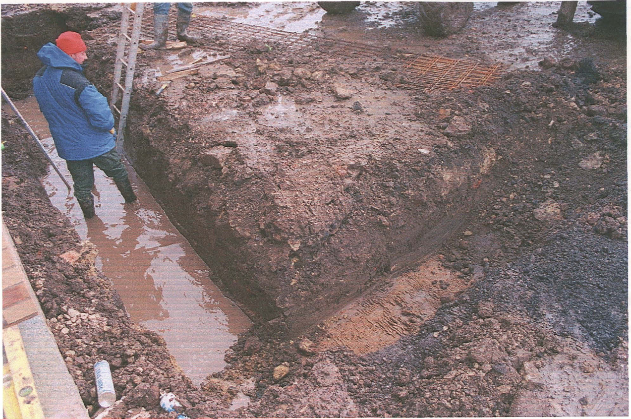
Pl.5 Excavation of garage foundations showing disturbed ground along east trench (right) and ingress of water
