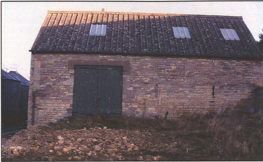
Pl. 1 Southern elevation of barn. Note revetted path leading up to double doors. Looking north.
