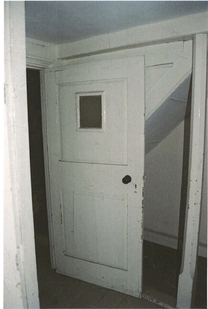
Pl. 7 Panelled door leading to inner first floor landing.
