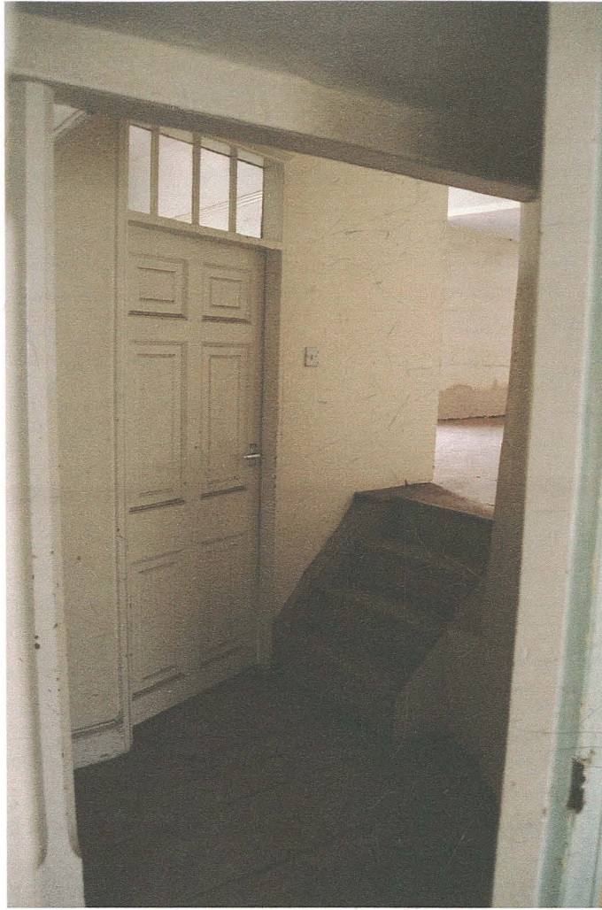
Pl. 10 First floor inner landing showing steps up to southern bedroom. Door to left of stairs leads to small front bedroom.
