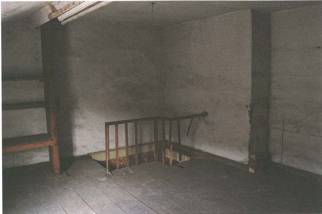
Pl. 12 Second floor rear bedroom, with stair in northeast corner.
