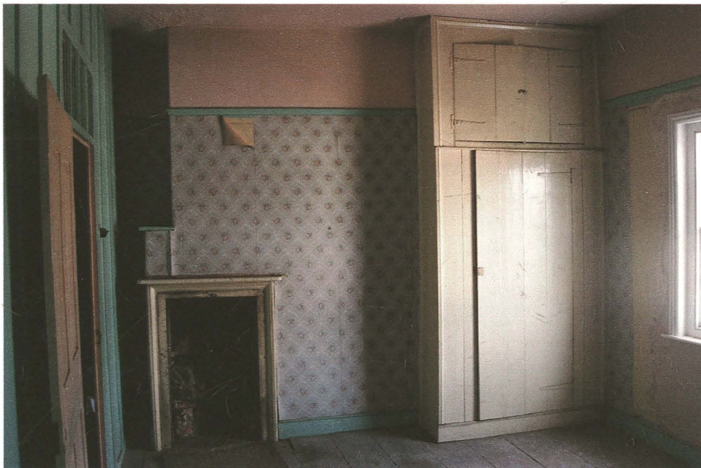
Pl. 17 Second floor middle bedroom. North wall with built in cupboard on east side of chimney stack. Note strap hinges.
