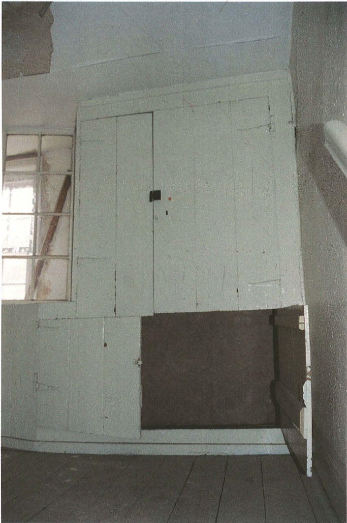
Pl. 6 Inserted cupboard on first floor landing. Note strap hinges and angled window providing borrowed light from sash window in bathroom.
