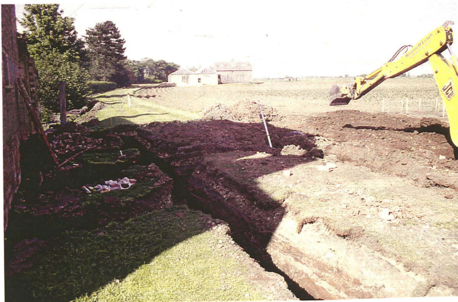
Plate 3 General view of the development area at completion of groundworks
