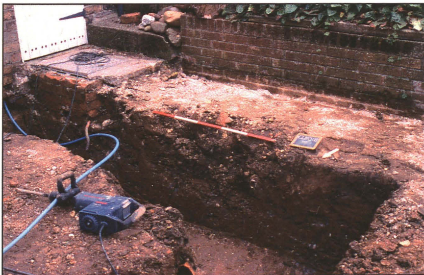
Plate 7: The south side of the completed foundation trench, looking SE.
