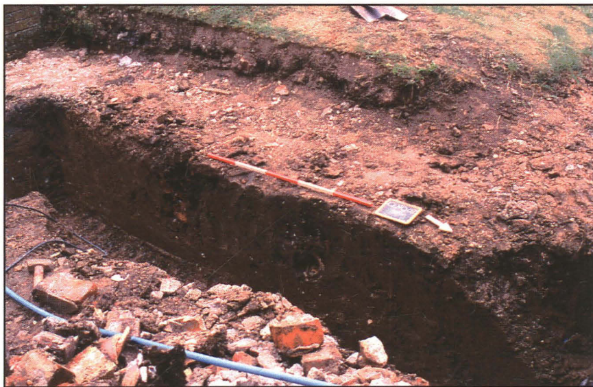
Plate 5 (above): Working shot during excavation, showing the difference in height between the house platform and the adjacent field, looking SE.
