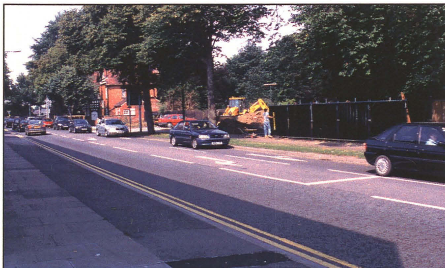
Plate 3 (left): General shot of the development site, looking north-east across Wragby Road.
