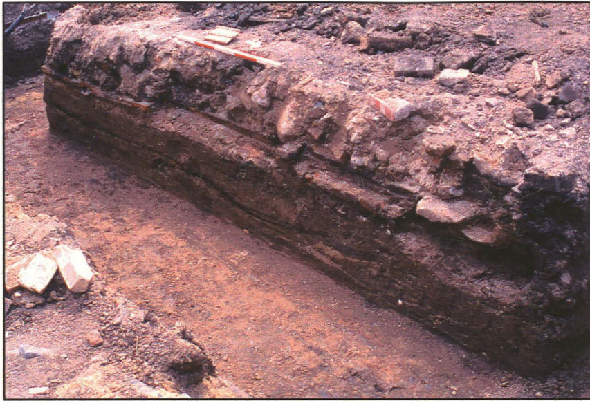
Plate 4 (left): Section of the south end of the foundation trench for the east wall of the new building, looking south-west.
