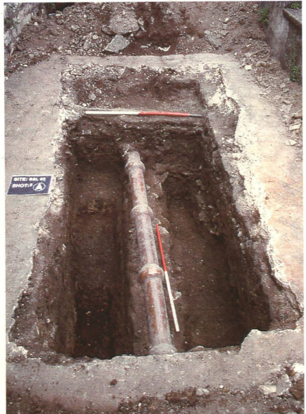
Plate 3 North facing view, showing evaluation trench during final stage of excavation.
