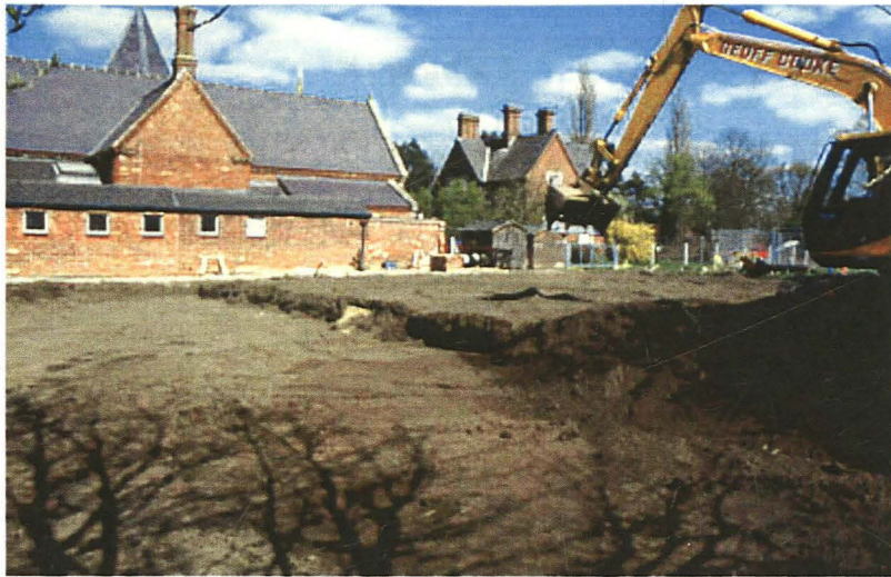
Plate 1 - General view of the development area, looking northeast
