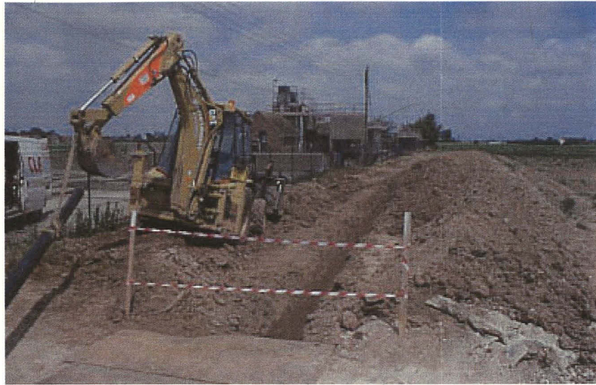
Plate 1 - General view showing the works in progress
