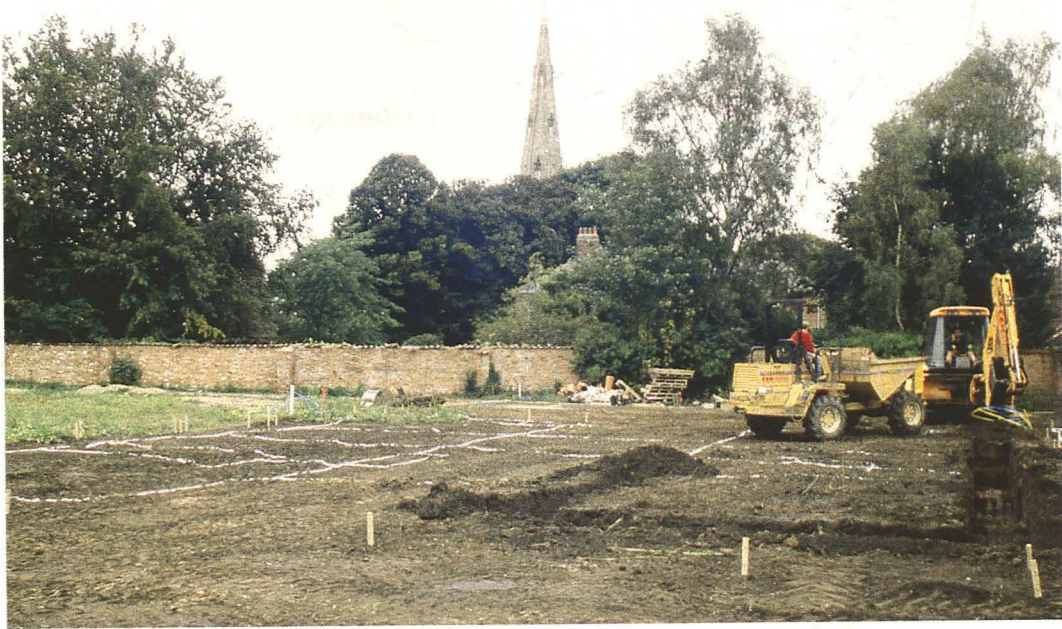
Plate 1 General view of the development area, looking north
