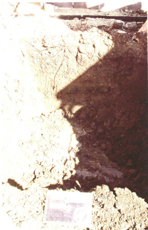
Plate 2 Soakway, Section 1, looking northwest
