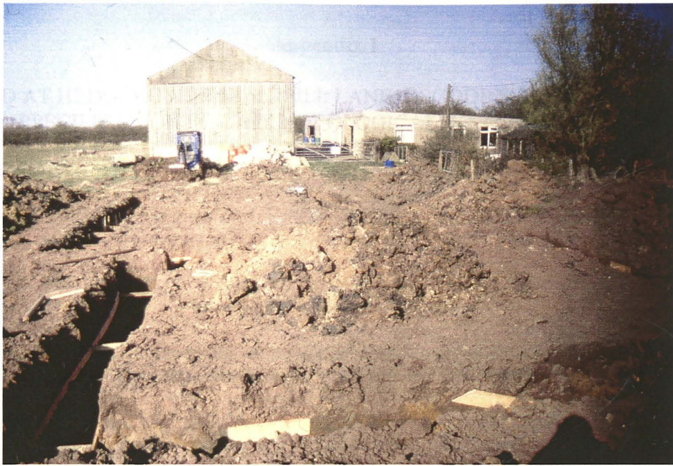
Plate 1 - General view of the development area, looking west
