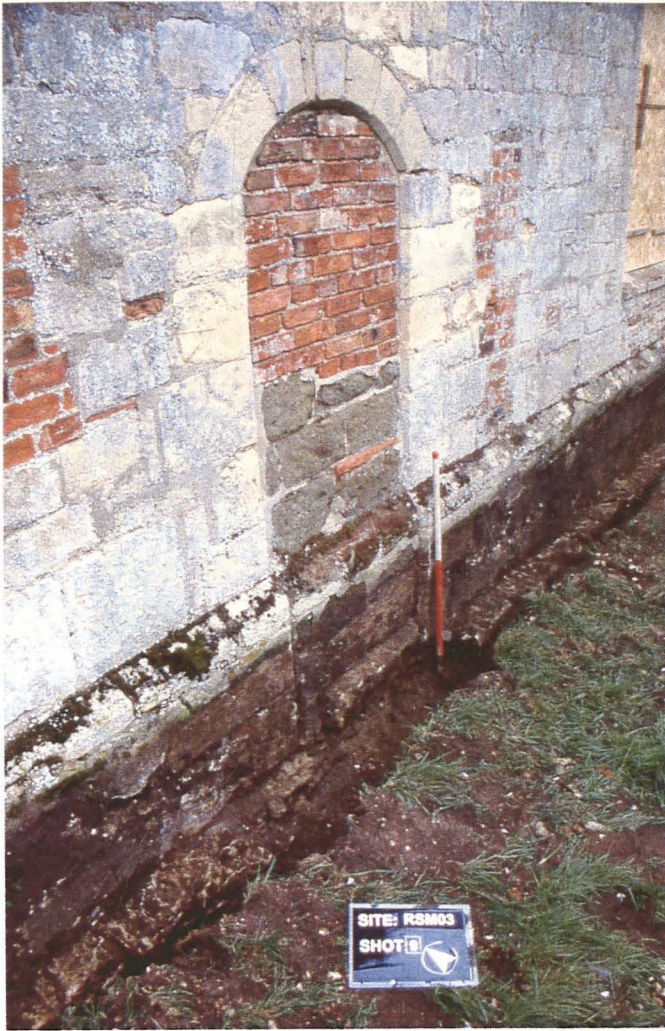
Plate 4 Blocked doorway in the south wall of the nave.
