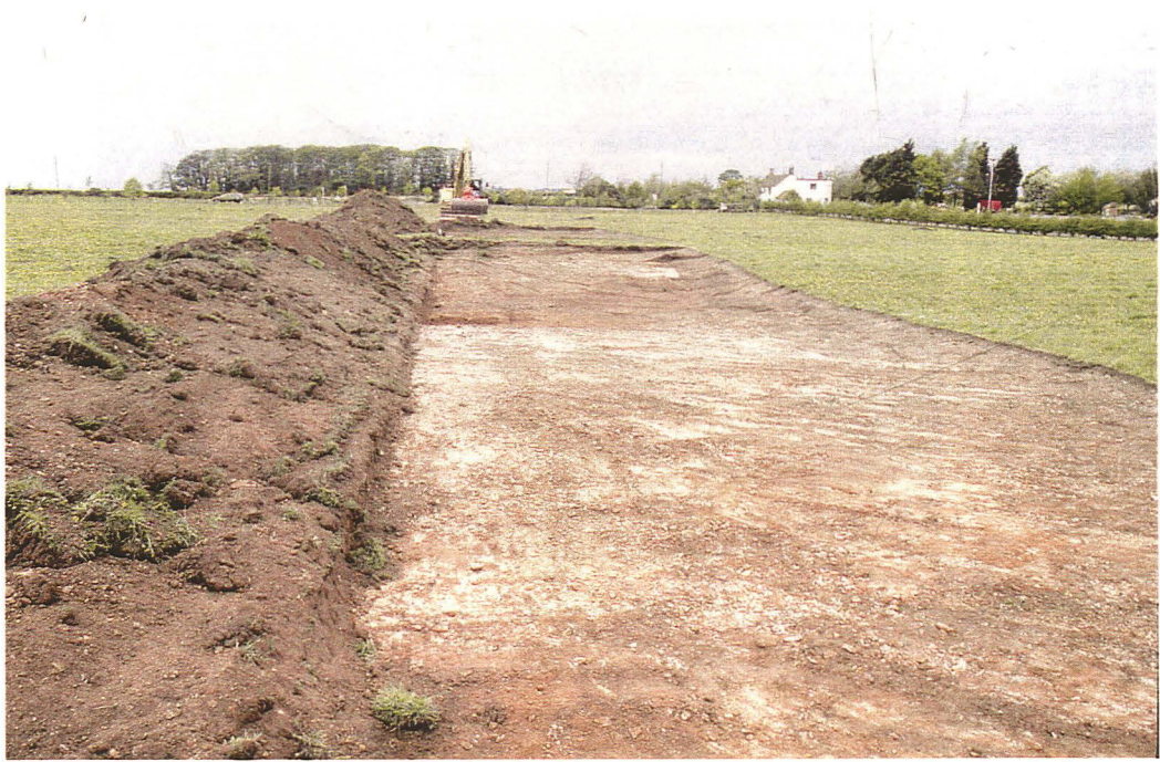
Plate 1 - General view of the site, looking west
