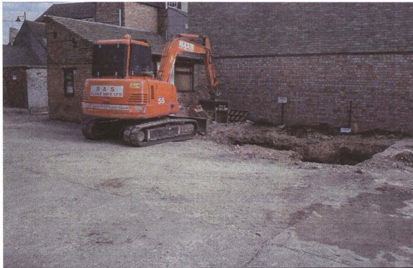
Plate 2: South facing view across site upon completion of machine excavation
