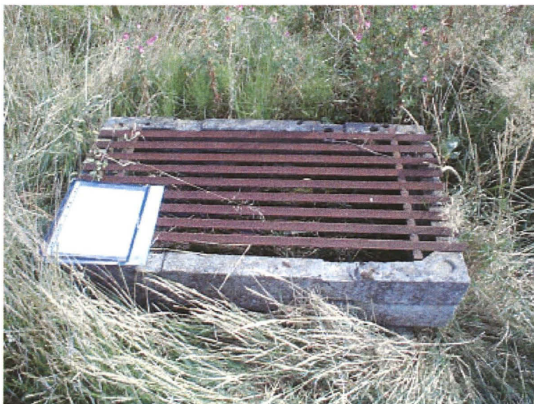
Plate 3 - The manhole cover located centrally in the field
