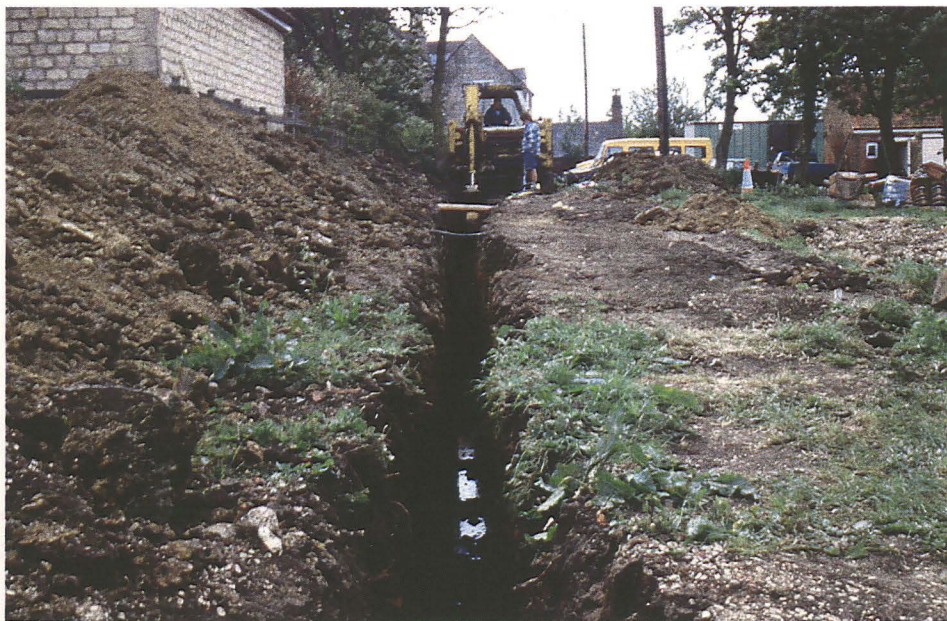
Plate 3 General view along east-west service trench
