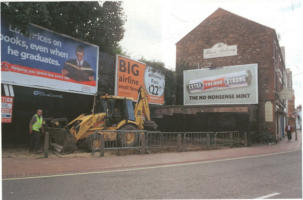
Pl. 1 Location of the evaluation trench. Looking south-west.
