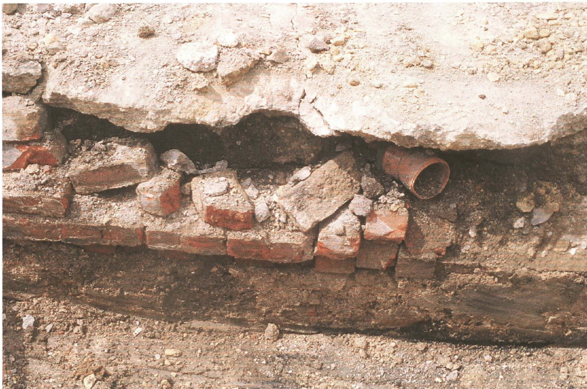
Pl. 6 Modern brick foundations located adjacent to the boiler house.
