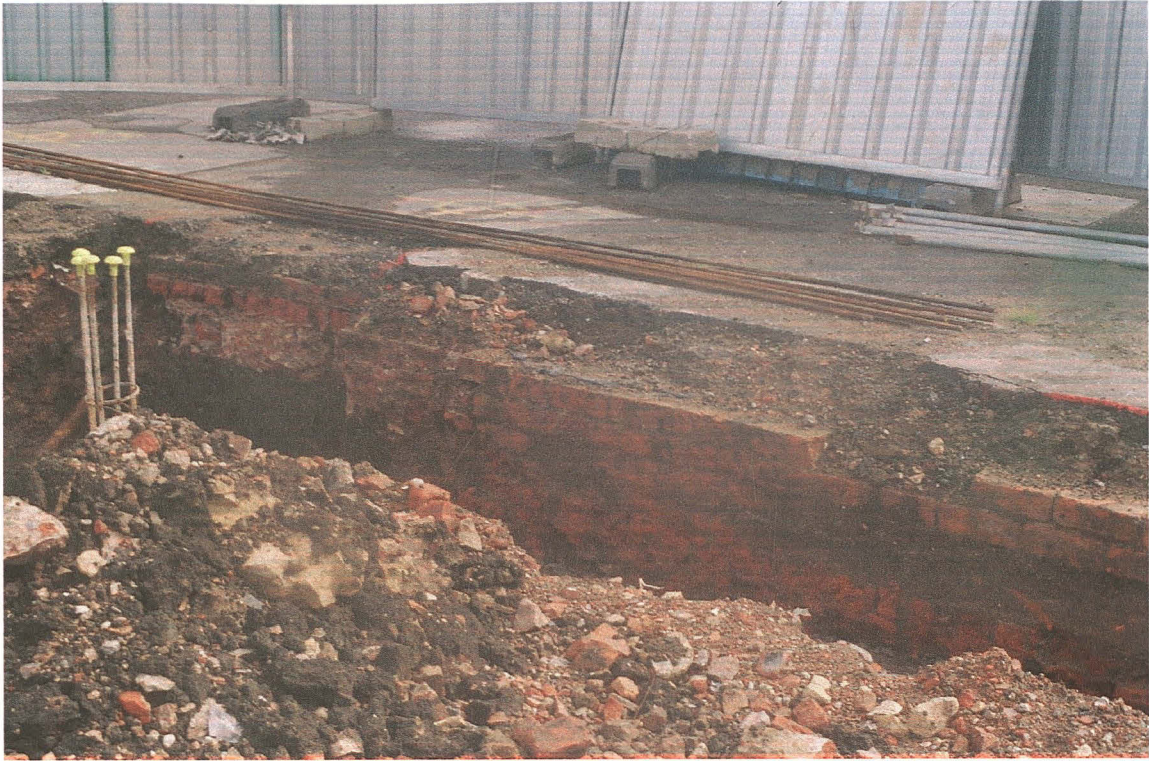
Pl. 5 Modern disturbance and 19th century foundations located immediately adjacent to Weir Street
