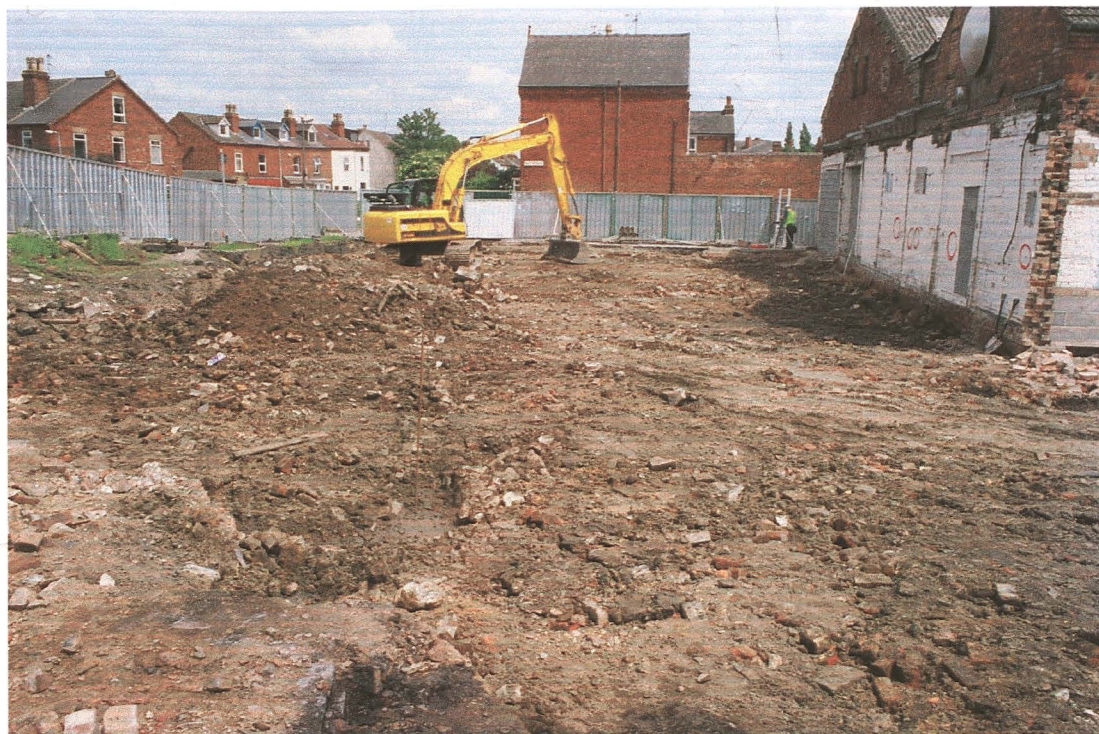
Pl. 3 General view of the site after stripping and lowering
