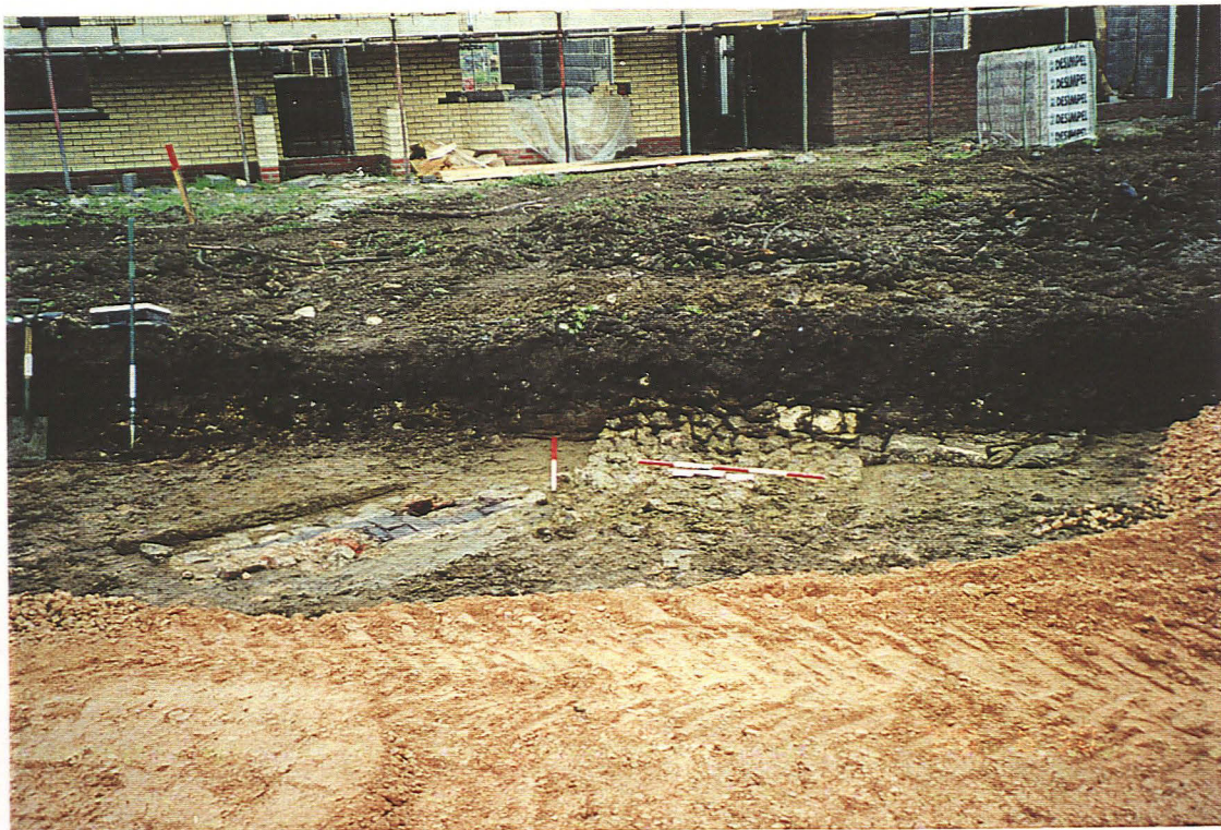
P10. Brick hearth (322) and stone walls (323) and (324); exposed in phase I access road, looking south
