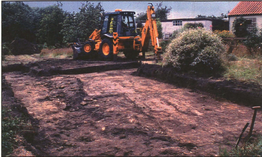
Plate 1: General shot of site with JCB at work, looking SW.
