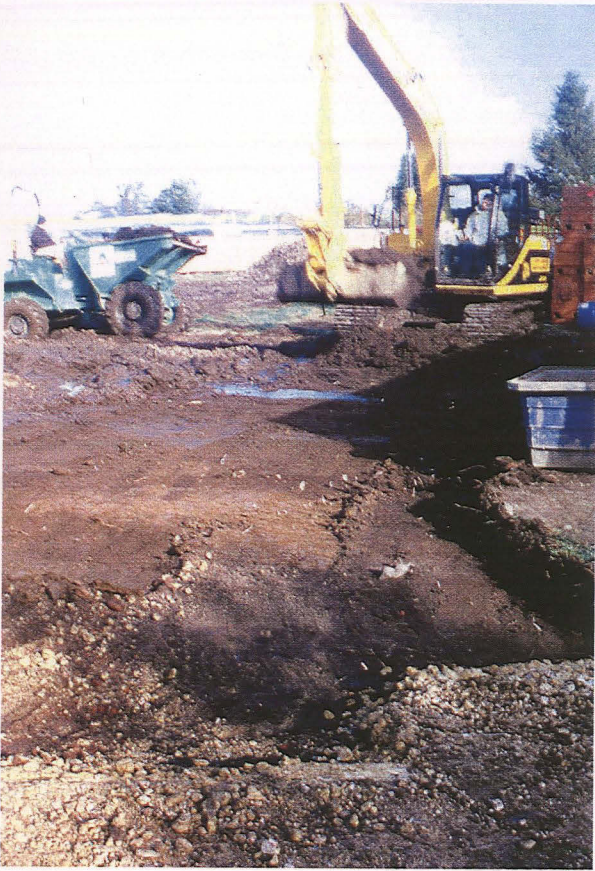
Plate 1 View of access road stripping in progress, looking north
