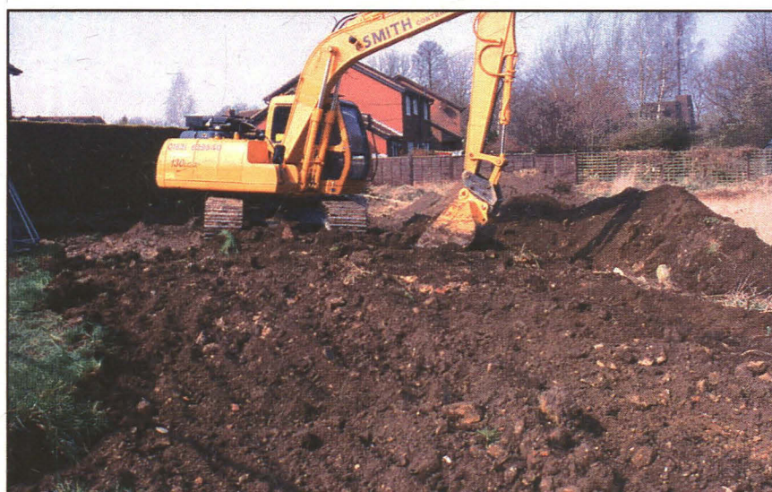
Plate 2 (right): General view of the site during topsoil stripping, looking north-west.
