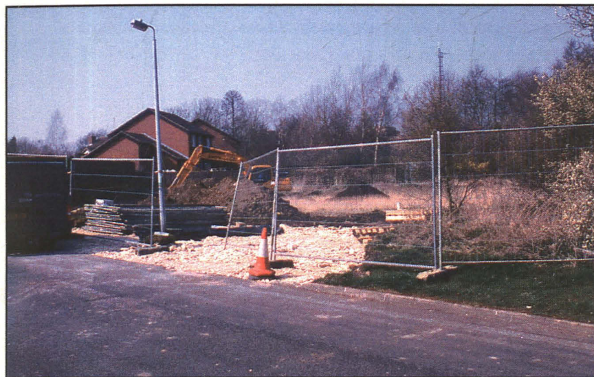
Plate 1 (left): General view of the site during machining, looking north-west.
