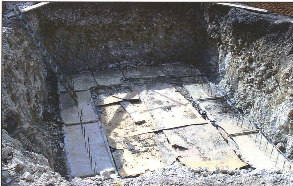
Plate 2(right): General view of the development site, showing the pit excavated for the cellar, looking east.
