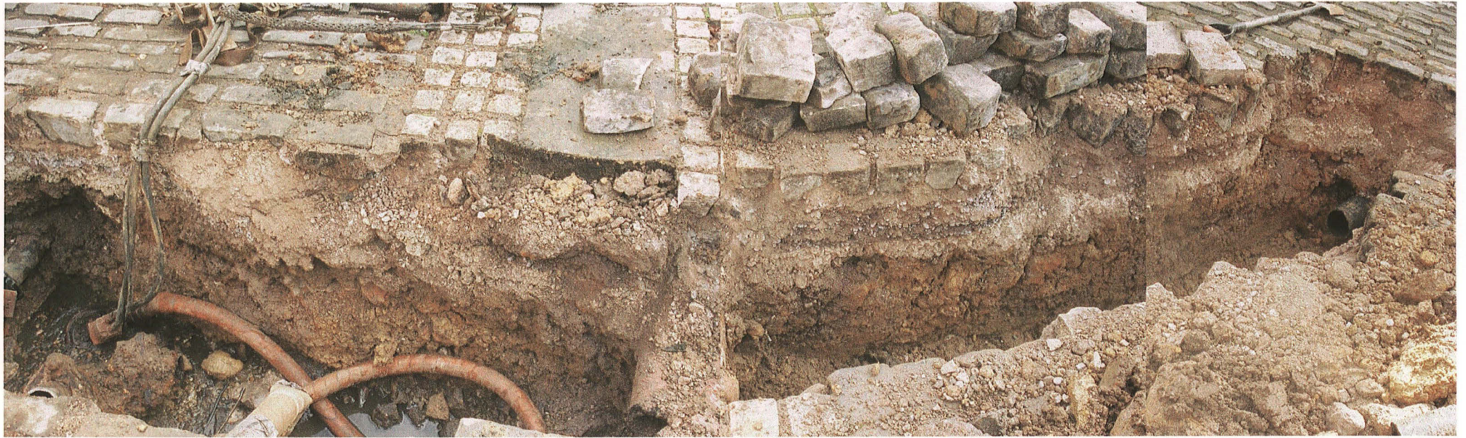
Pl. 17 Composite photograph showing deposits in the SE trench face at 20. Note the dark clay below the double ceramic pipe, thought to be ditch fill with apparently undisturbed clay to the right (looking SE at the junction of Michaelgate and Steep Hill).
