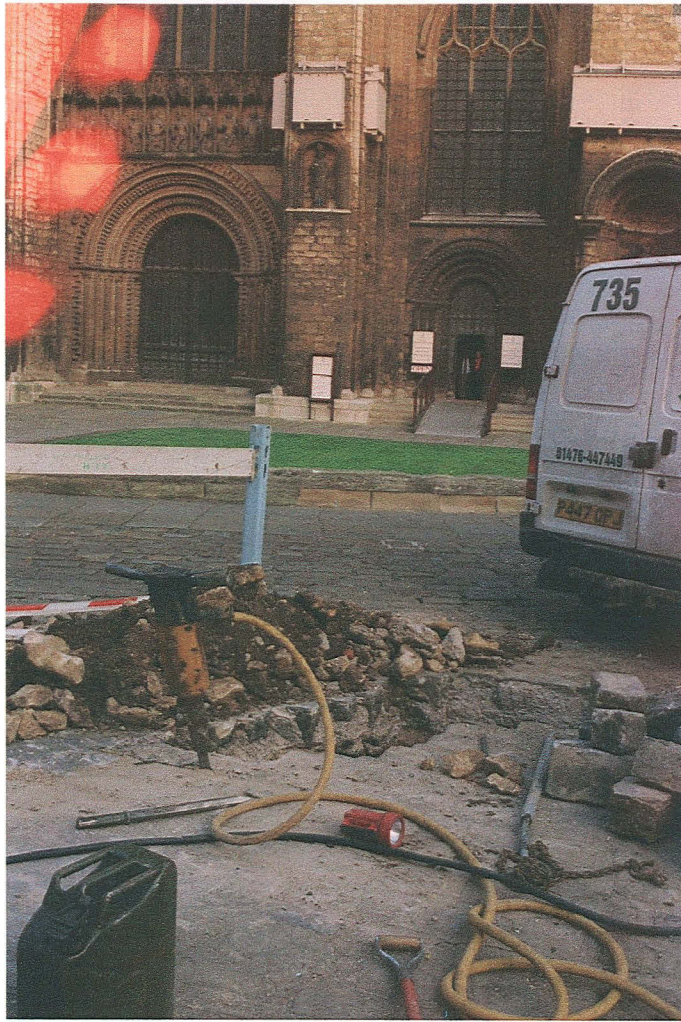
Pl. 13 Position of 16, in Minster Yard, east of Exchequer Gate (looking east).
