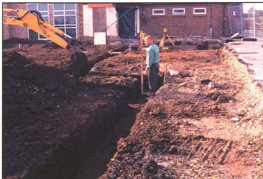
Plate 3 (right): Working shot, showing excavation of foundation trenches in the NE corner of the site with the rear of the school buildings behind, looking N.
