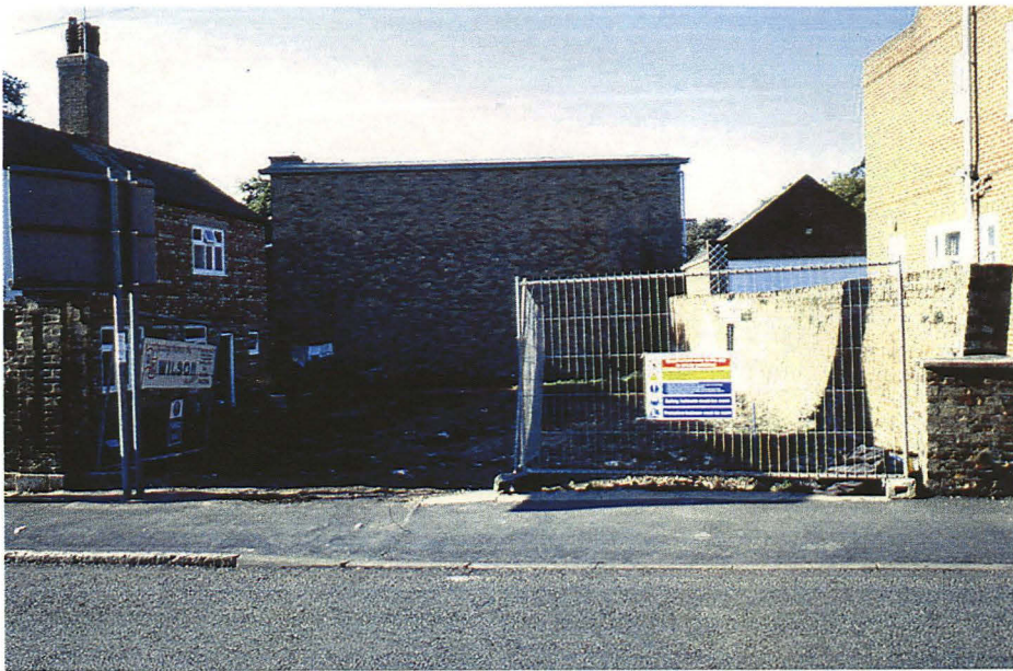
Plate 1 General view of site from Church Street looking south
