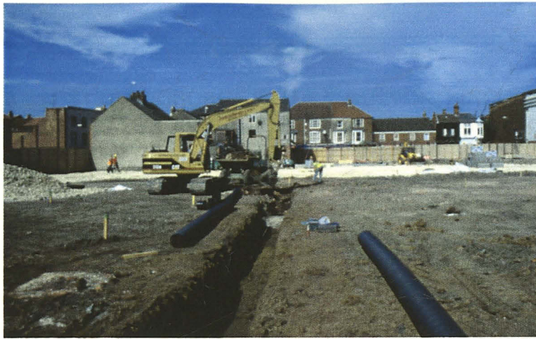
Plate 1 - General view of the drainage trench, looking north
