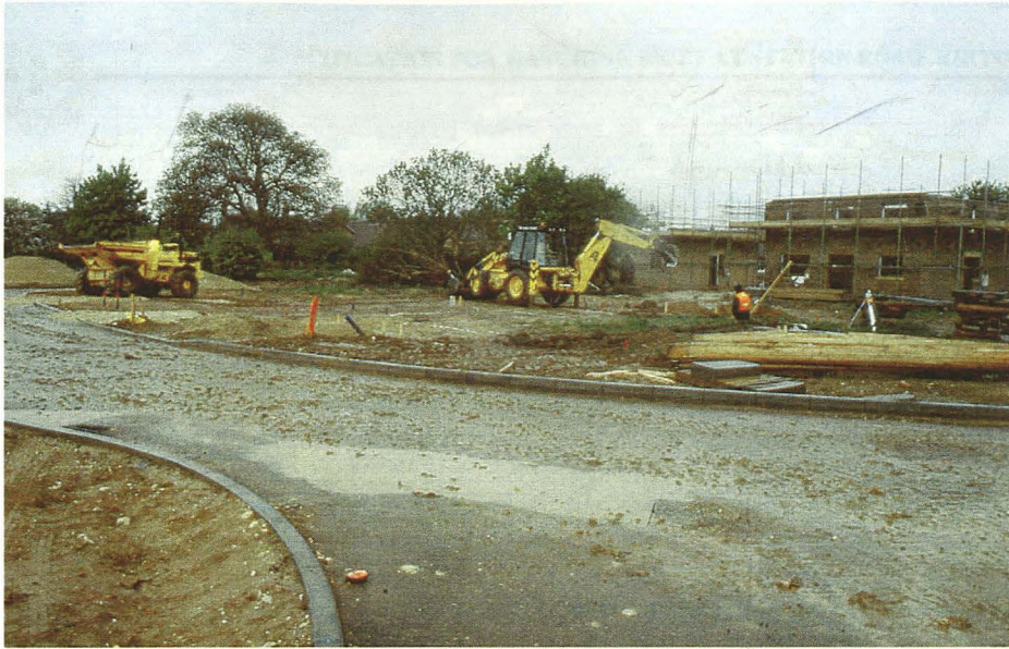
Plate 1 General view of development area, looking northwest
