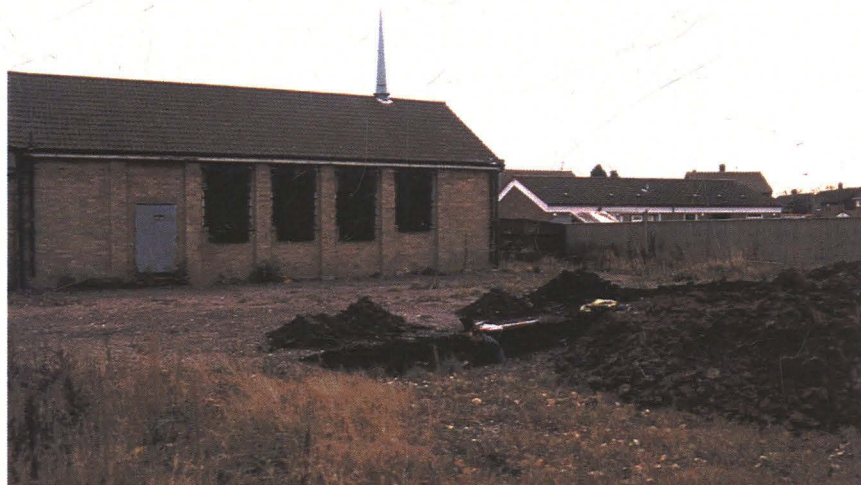
Plate 4: General view of the rear of the redundant Congregational Church showing the location of Trench 2, looking south-east.
