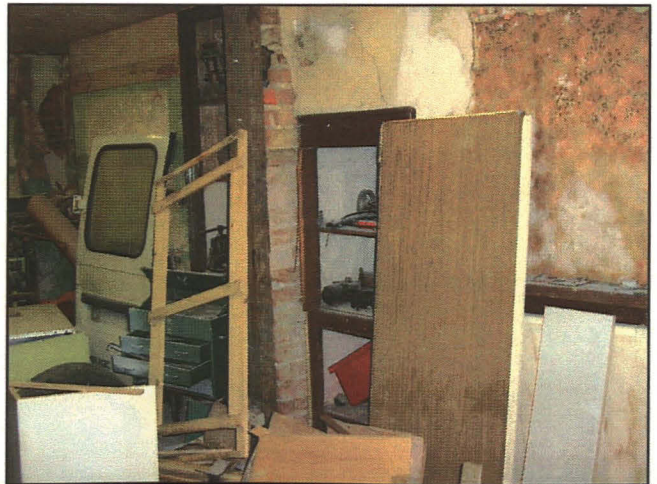
Plate 15 (right): Interior view of room 1 in building 1, looking NW.
