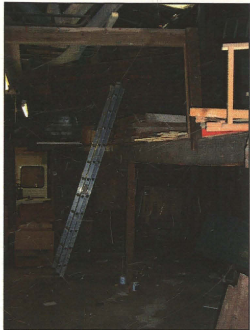
Plate 13 (above): Interior view of building 2, looking north.
