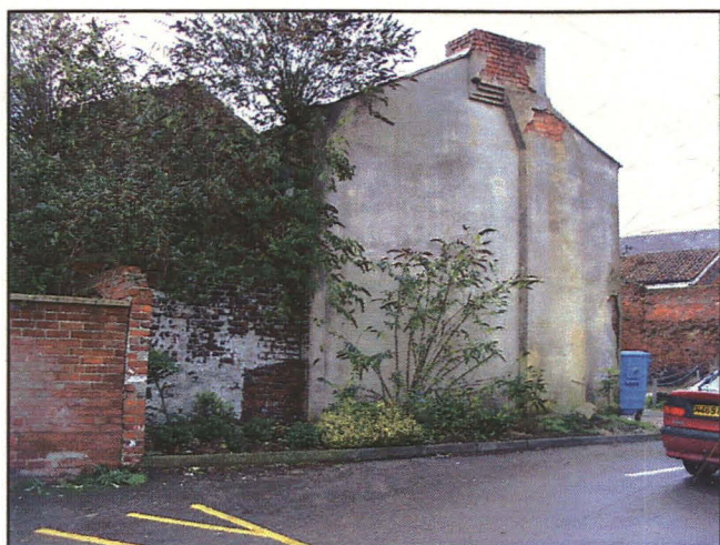
Plate 4 (left): General view of the north elevation of building 1, looking SW.
