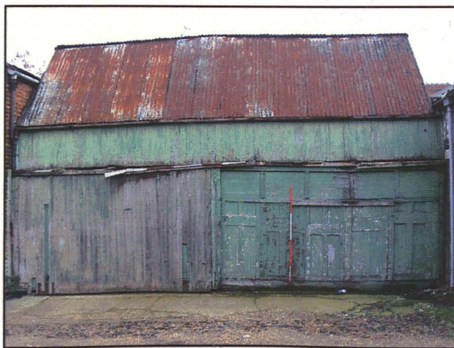
Plate 7 (right): West facing elevation of building 2, looking east.
