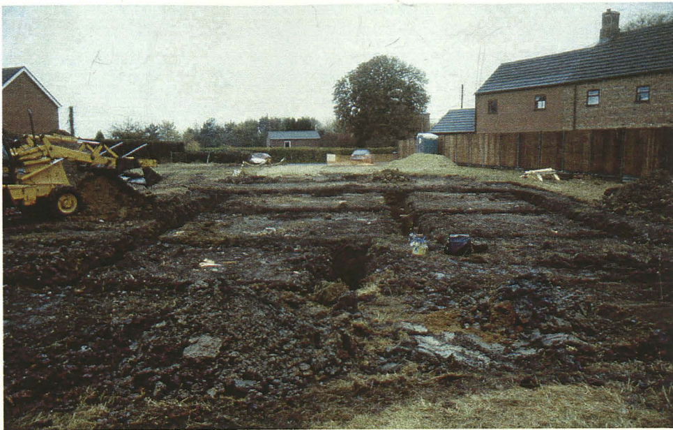
Plate 1 General View of Site looking South
