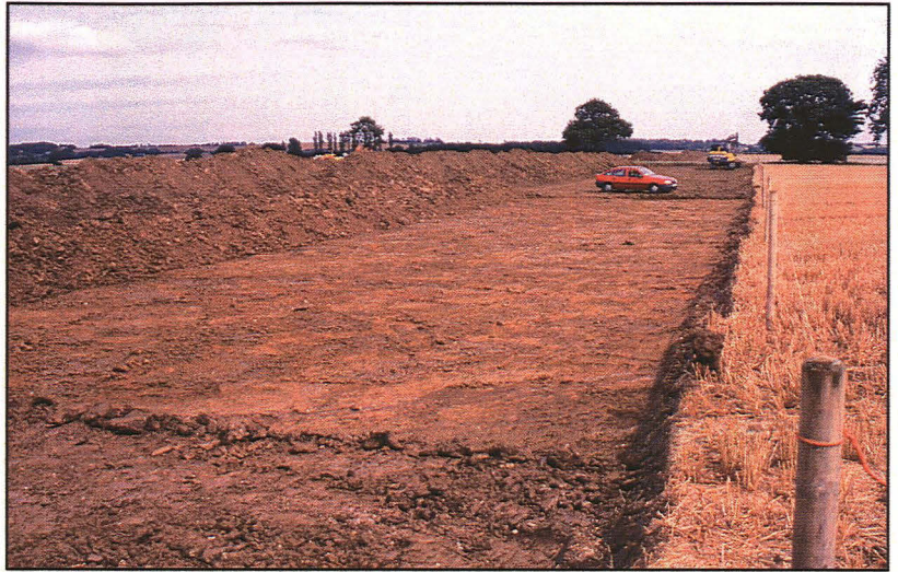
Plate 10: General shot of Site 3 after machining, looking E.
