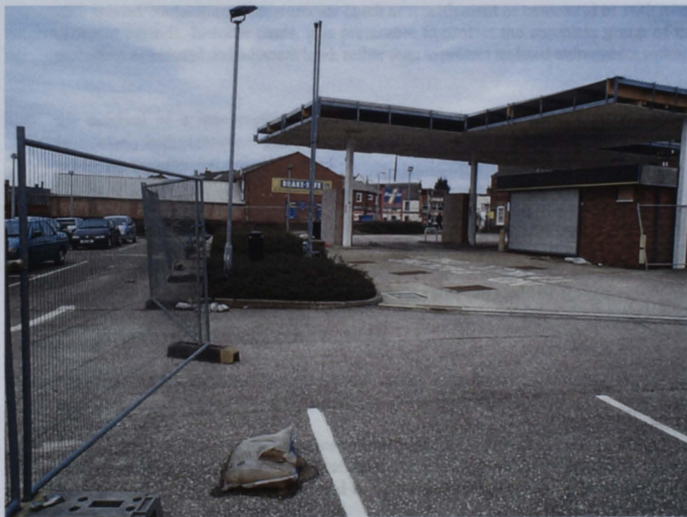
Plate 2 - The proposed development area from the northwest. In the foreground are the manhole covers believed to be associated with the buried fuel tanks. Vent pipes are visible in the centre of the picture along with a lamppost.
