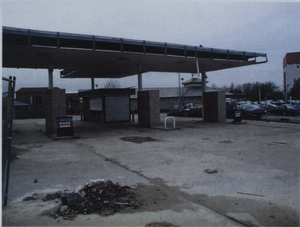
Plate 1 - View of the proposed development area from the southeast of the site showing the kiosk, canopy and pumps. Also visible are the trial pits and borehole taken across the site.
