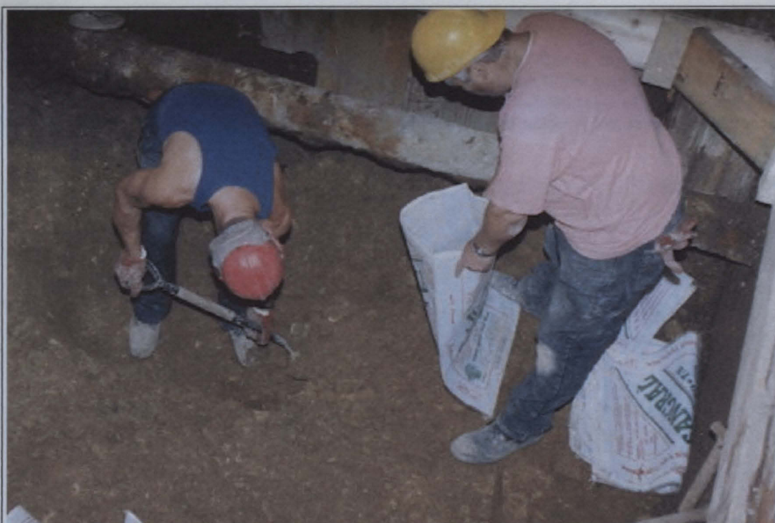
Plate I: General view showing the manual excavation of Lift pit B.
